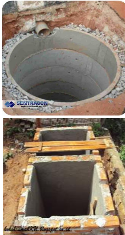
Figure 1. Septic Tank Concrete & conventional
