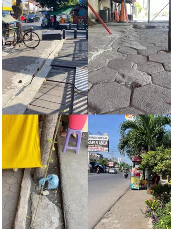
Picture 1. Existing Condition of the Sidewalk
