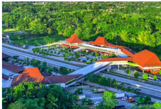
Figure 3. Pendopo Rest Area KM 456 Source: astraproperty.co.id, 2026
